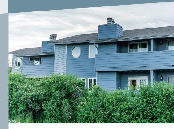
The Baywatch Condominiums in Homer, AK, is a beachside property in coastal Alaska originally constructed in 1980. On the exterior, the structure featured T1-11 wood siding that failed due to consistent exposure to sun, wind, and moisture from the sea. The owners, Baywatch Condominium Association, were looking for a solution that solved the performance issues of the failed wood siding and would enhance the building's overall appearance.
