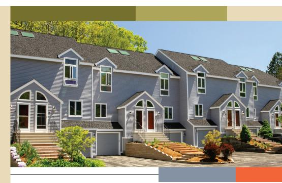
Hager Meadows is a 10-building, 84-unit condominium complex located in Marlborough, MA. The homes were built in 1988 with an exterior that was constructed of low-grade cedar siding, a material that breaks down after yearly freeze-thaw cycles in climates such as the one in Massachusetts.
